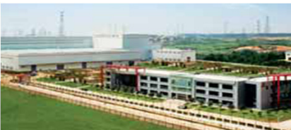
Wuhan, China The world's first power transformer factory to receive green certification
