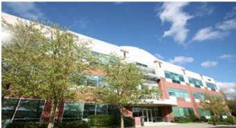
Redmond, USA Network Management Systems
