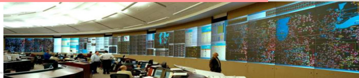
Network Management Systems Digital Control Systems
